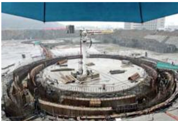
China's Fangjiashen nuclear power plant during construction // Source: energytribune.com
