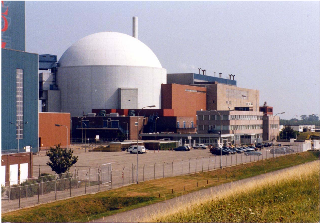
Borssele Nuclear Power Plant
