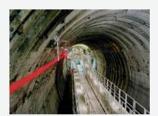
Rear of boring m a c h i n e showing laser guidance system // Source: agiweb.org
