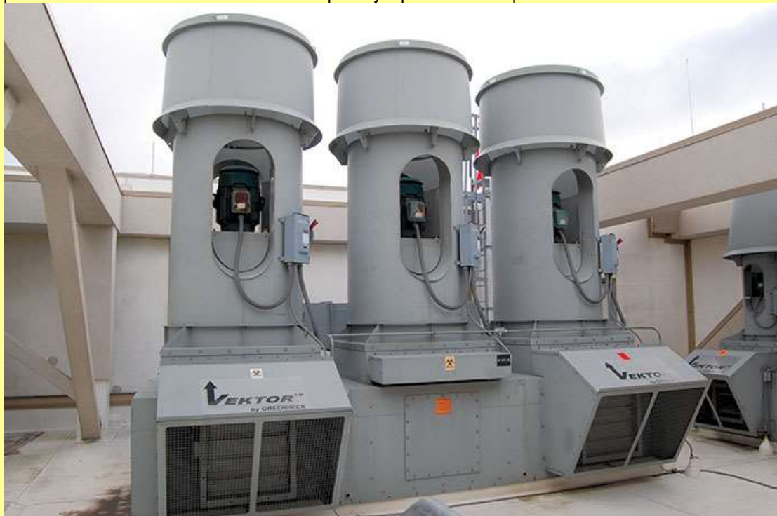
The exhaust fan should be located outdoors and placed as far away from intakes and public areas as practical with discharge above the roof. Image courtesy of RTM Engineering Consultants
