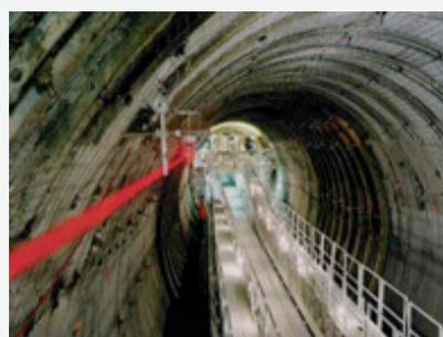
Rear of boring machine showing laser guidance system // Source: [agiweb.org](http://agiweb.org)
