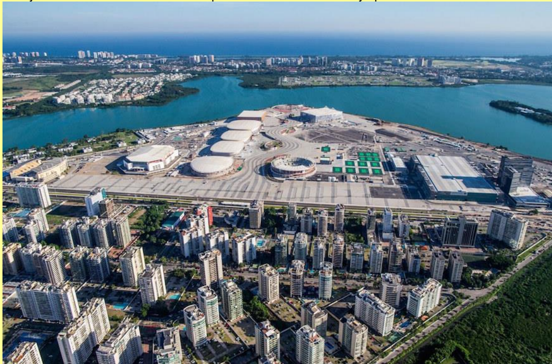
An aerial view of Rio 2016 Olympic Park during construction ( Gabriel Heusi/Brasil2016.gov.br )
