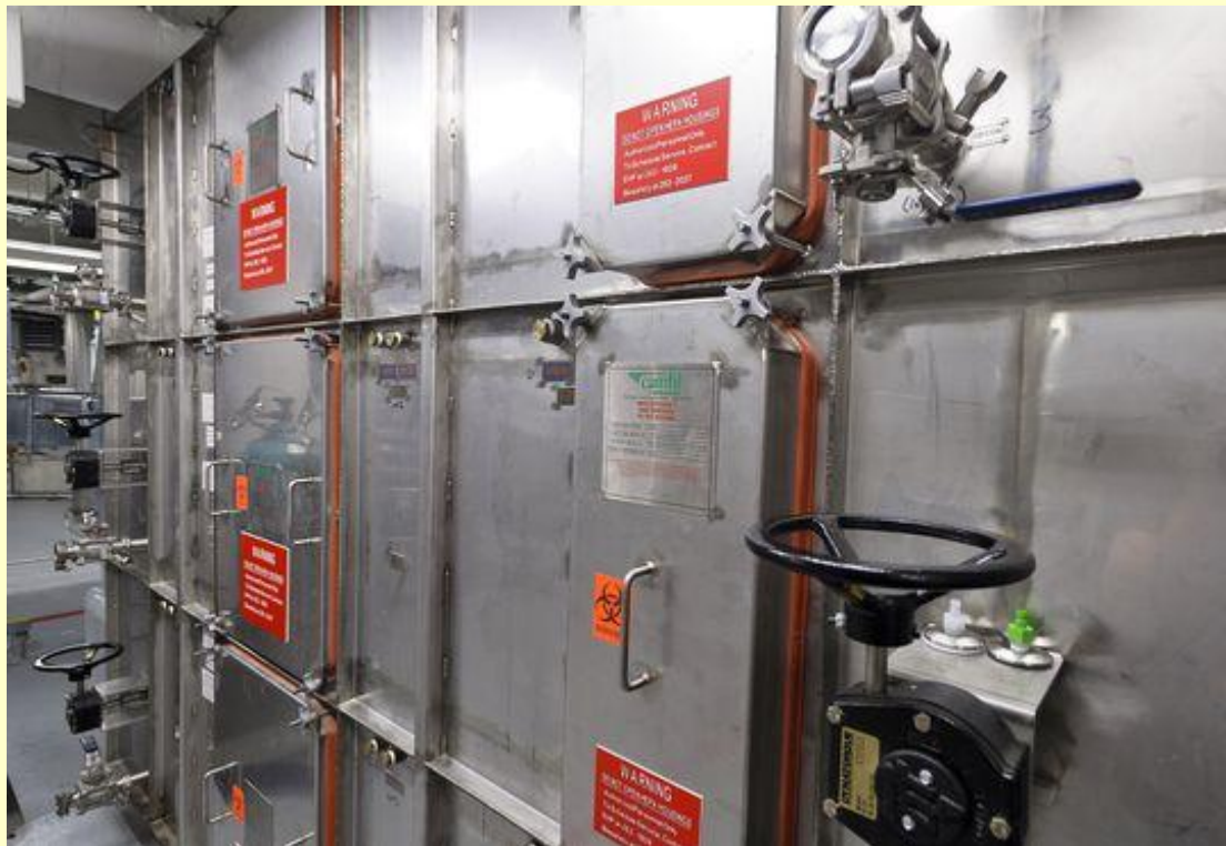
A ventilation system designed to filter the building's air supply through a series of HEPA filters is seen during a tour of the Influenza Research Institute at the University of Wisconsin-Madison on Feb. 13, 2013. (Photo: Bryce Richter, University of Wisconsin-Madison)
