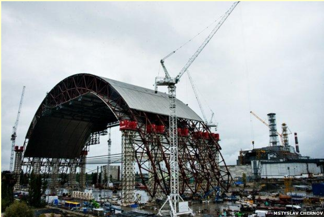
The ends of the arch will also be sealed
