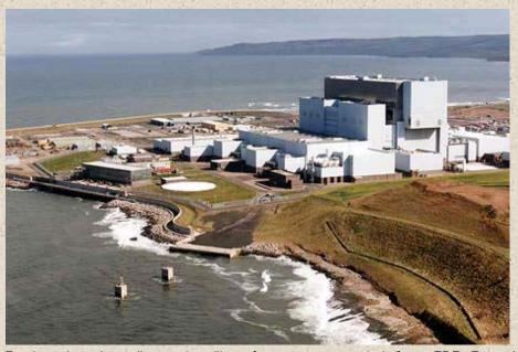
Reactors but also relies on supplies of sea water to ensure it operates safely. It has filters which are designed to prevent seaweed and marine animals entering the cooling system.
