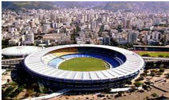
Maracanã stadium in February 2009, showing the two-tier configuration and concrete roof
