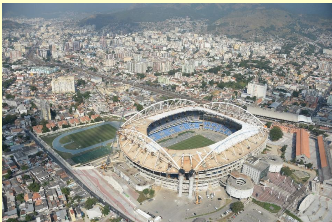
Aerial view of the Nilton Santos Olympic Stadium under construction for the Rio 2016 Olympic Games, taken on July 28, 2015 (AFP Photo/Vanderlei Almeida)
