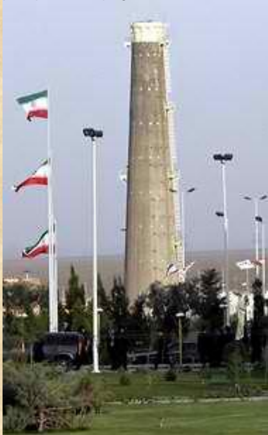
Iran's nuclear enrichment facility at Natanz.
